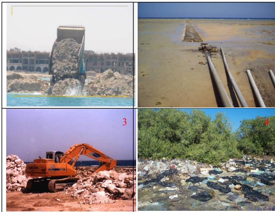
Plate 3: 1) Landfilling processes at Hurghada, 2) Reject pipeline from the desalination and power plants, 3) Dredging operation inside Hurghada, and 4) Solid waste disposal at Quiah locality.
