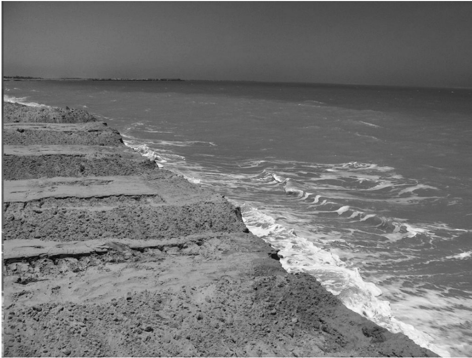
Fig. (10): Sand nourishment along the eastern zone of Marina center.
