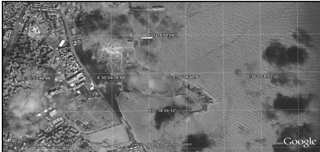
Figure 3. El Tabia Pumping Station
